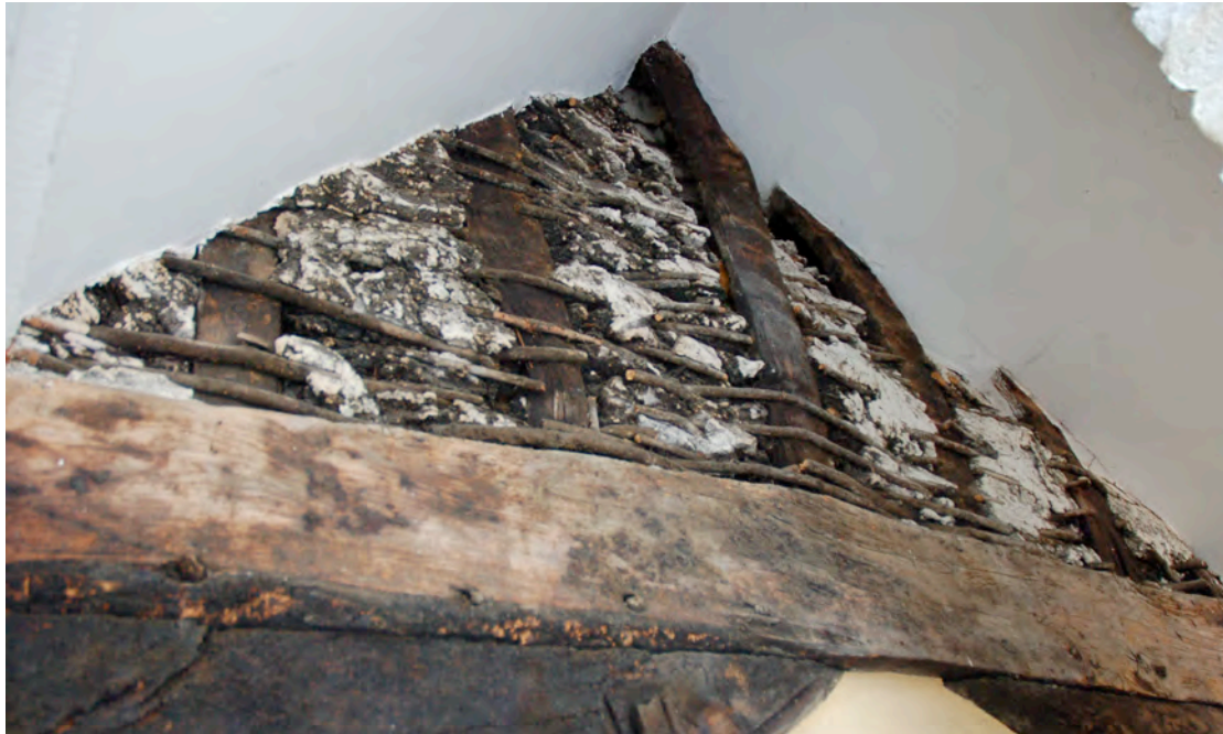
The truss beam plus wattle and daub
