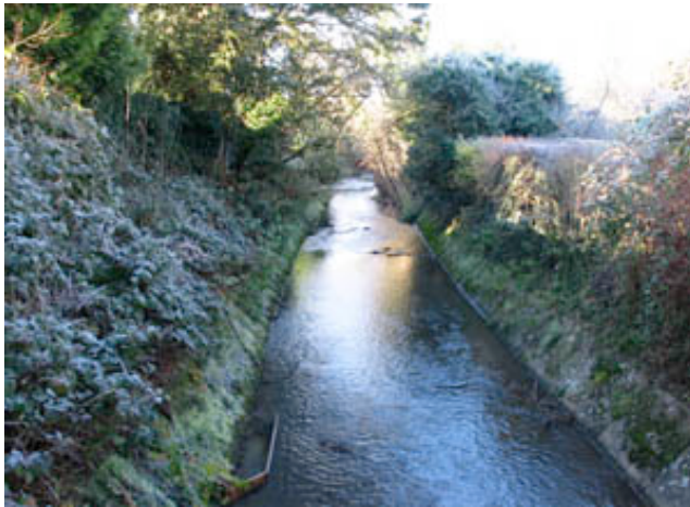
The new culvert west of The Cross
