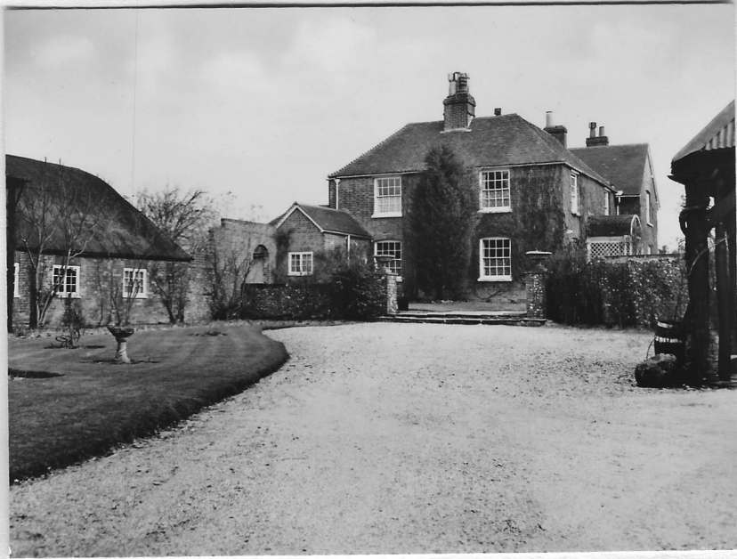
COOMBE CROSS HOUSE.
