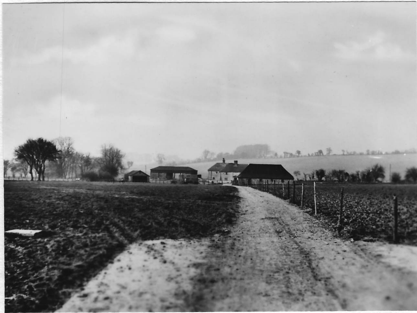
LOWER PEAKE FARM BUILDINGS AND COTTAGES.
