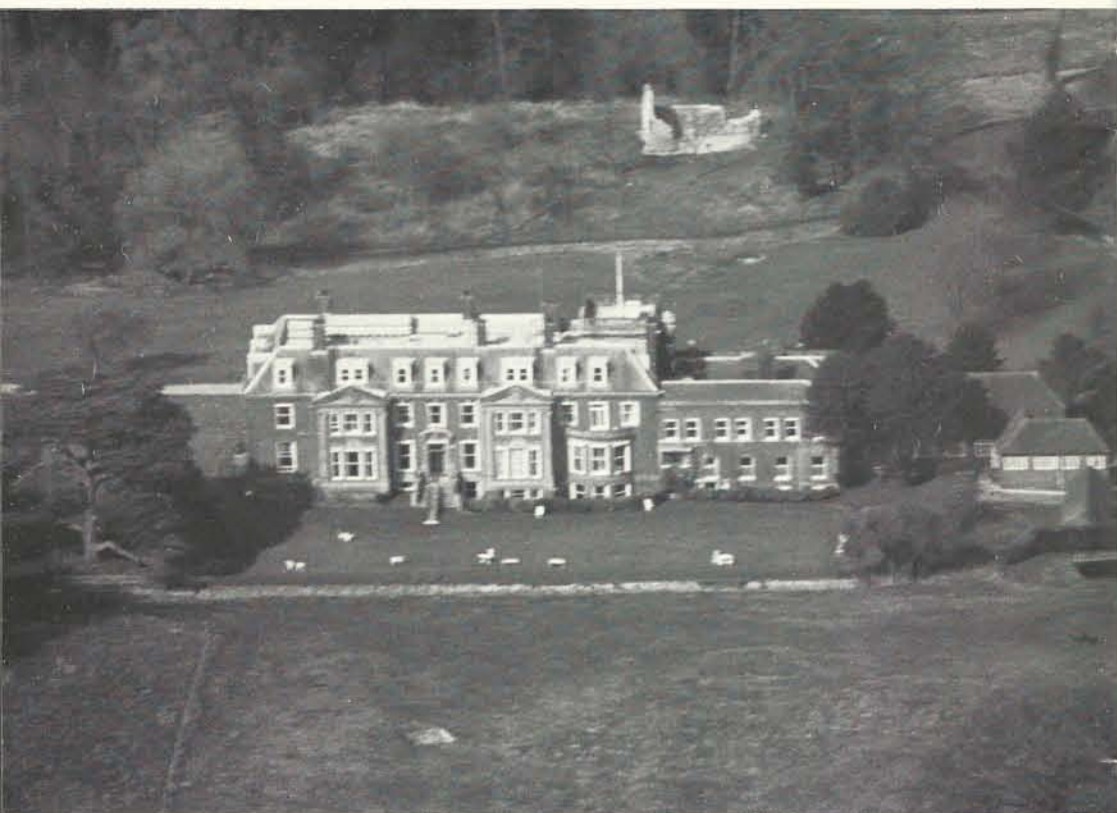
House and Grounds as seen from the air. The Chapel Ruins, on the North Side of the River Meon, have the East Meon road just beyond them. The Lake is to the East.
