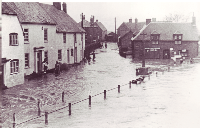
Barnards during 1952 flooding – Hazel Goddard, now Pamplin, on the doorstep.
