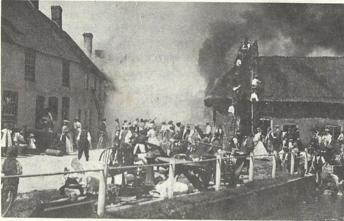
Fire at East Meon 1910 at what is now Mr Witts shop and showing old Barnards Cottages.
