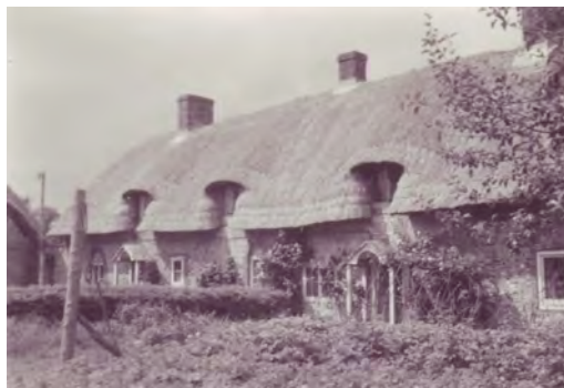
Cottages in Workhouse Lane, now named Kews and Paupers.
