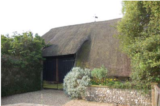
Fig 3 The 17 th century barn at The Court House, which probably replaced an earlier barn for the collection of crops harvested for the manor, or greater tithes, or both, in which case, they would have been kept strictly separate.
