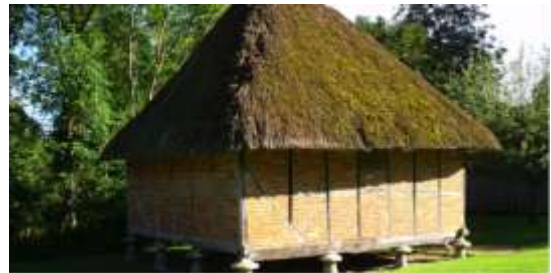
Granary from Weald and Downland. Grain stores were raised from the ground to exclude rodents.
