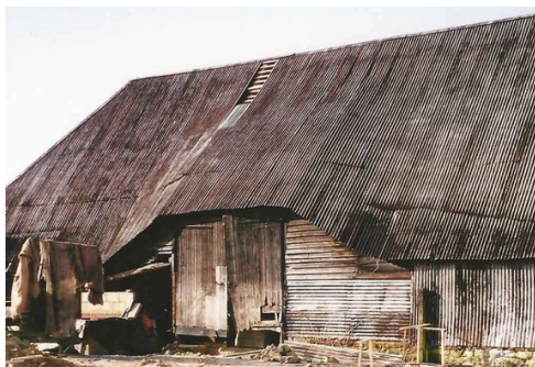
Upper Parsonage Barn before restoration
