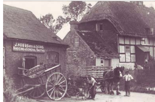
East Meon Forge, and Forge Cottage on right
