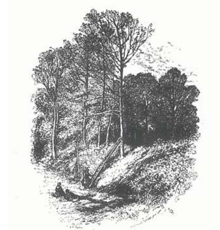
19 th century engraving of the embankment at Merdon Park
