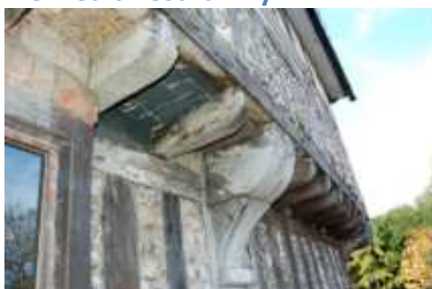
Fig 26 Jettying of first floor of Tudor House
