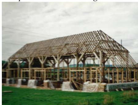
The frame was moved 30 metres to the south west ...
