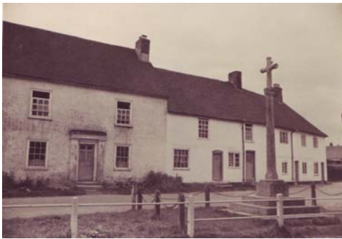
Fig 85 Five doorways at Barnards Corner at the turn of the century; there are three today
