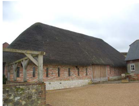
Fig 33 Upper Parsonage Barn, built c 1700, a 5-bay barn with central doors, 21.5 metres long, 8.5 metres wide, 5.2 metres high
