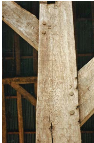
Fig 41 & 42 Masons' marks on posts and braces at Parsonage Barn
