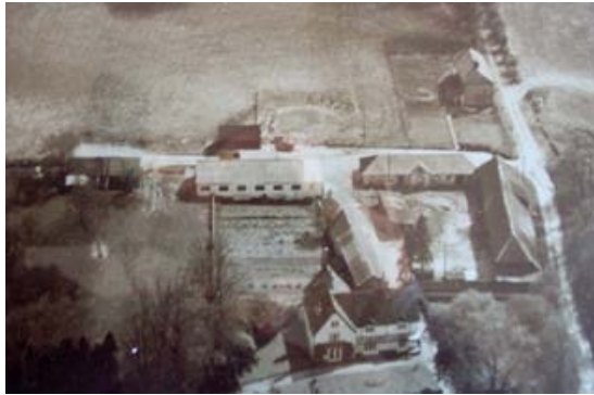
Aerial view before restoration, looking south, showing barn on right touching the cow house
