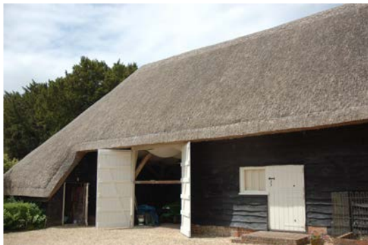
Fig 34 Oxenbourne House barn, c 1700, restored by its current owners. It is 12.8 metres long, 5.5 metres wide and has five bays
