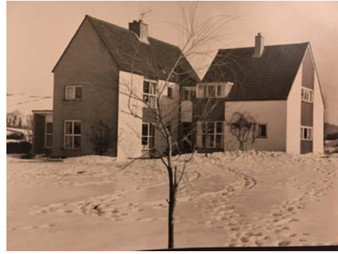
The new farmhouse built by Brian Blacker
