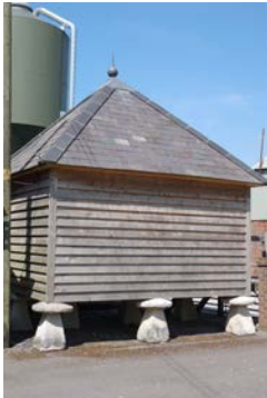
Fig 62 Granary on staddle stones at Hill Hampton Farm
