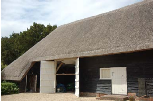
Fig 36 South entrance to Oxenbourne House barn
