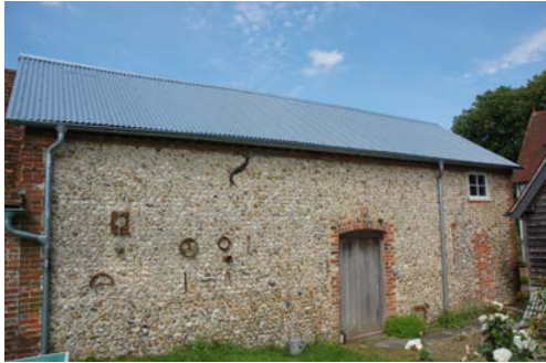
Fig 60 East wall of Lythe House stable
