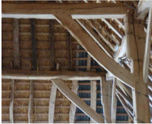
Fig 43 Convex braces at Upper Parsonage Farm
