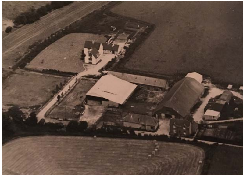
Fig 96 Photograph of Garston Farm, 1960
