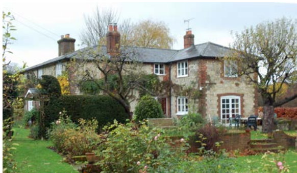
Fig 78 The north- eastern extension
