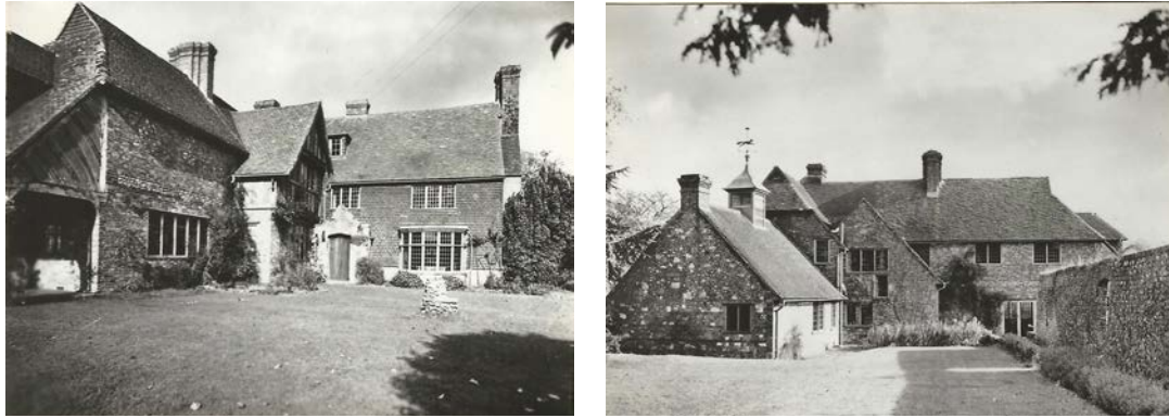
Figs 87 & 88. Photographs from Leydene Estate Sale, 1953 Now named Oxenbourne House , it had been substantially altered by Geoffrey Lupton , a prominent member of the Arts and Crafts movement .
