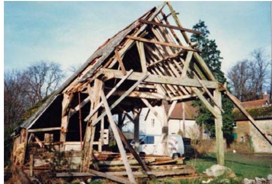
Lythe House barn before restoration work began
