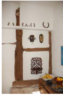
Figs 82 Lythe House: only these beams remain from the 17 th century structure
