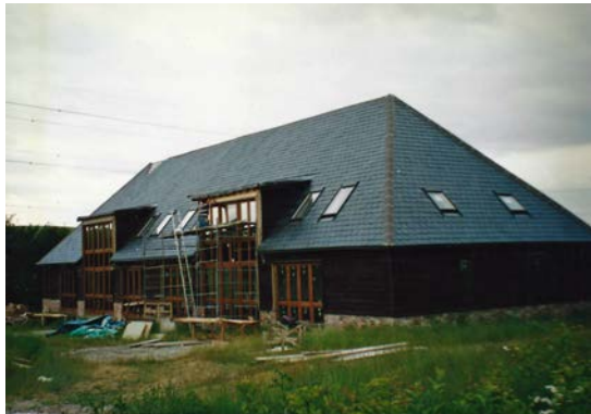
Fig 32 Parsonage Barn, a house built around the frame of a 17 th century barn. It was 25 metres long, 9.3 metres wide and had two sets of doors..
