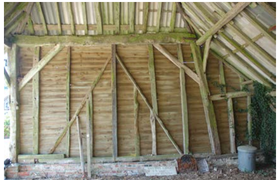
The barn's south wall restored as it had originally been
