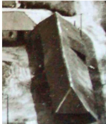
Fig 39 Aerial photograph of Lythe House barn before collapse and restoration
