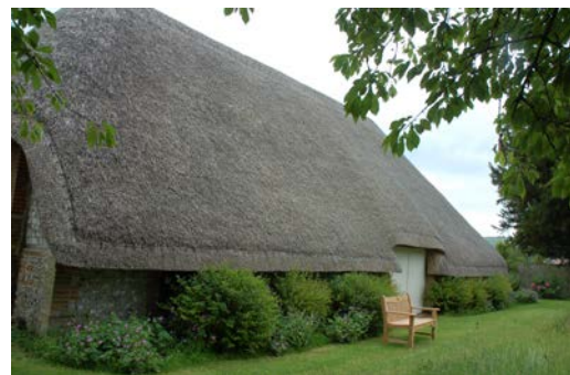
Fig 46 Aisle and west door of Oxenbourne House barn
