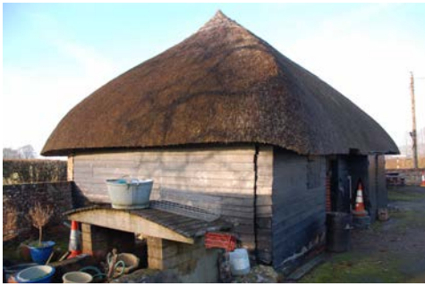
Fig 68 Cartshed at Lower Farm, entrance angled to avoid sunshine
