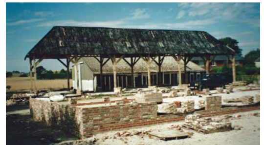
Parsonage Barn stripped down to its skeleton
