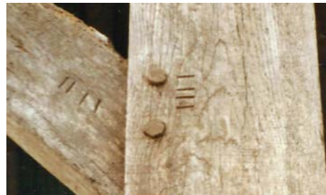
Fig 41 & 42 Masons' marks on posts and braces at Parsonage Barn
