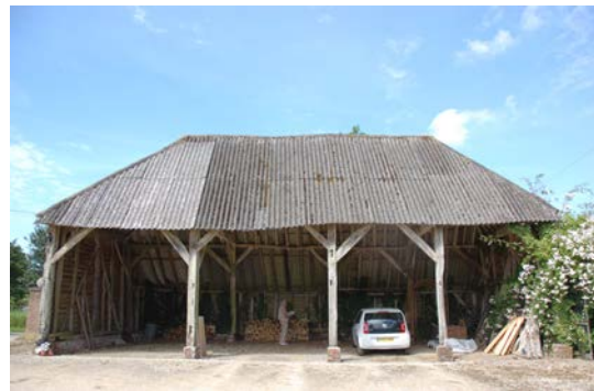
Fig 35 Lythe House barn, built c1800, was rescued from dilapidation in the 1960s. the current building is 12.8 metres long, 7 m. wide
