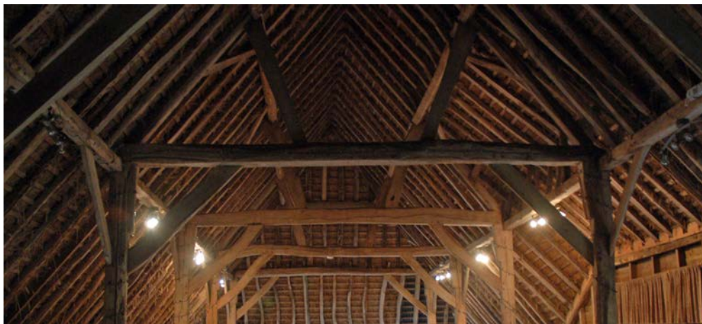
Fig 44 Upper Parsonage barn showing central arcade and aisles
