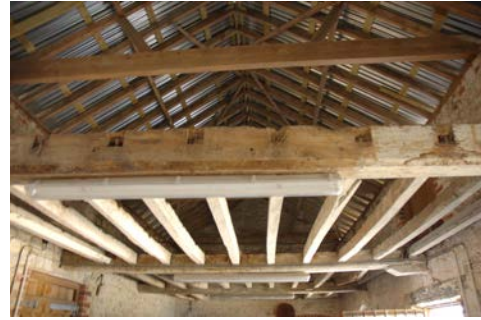
Fig 61 Lythe House stable ceiling timbers
