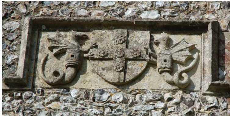
On the outside east wall, the rebus of Bishop Langton
