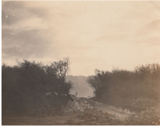
Cutting out the new road March 1922
