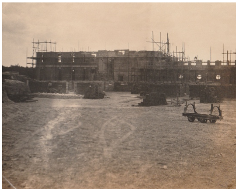
N.W. Angle showing Bull's Eye Windows under Batchelor's rooms August 1922
