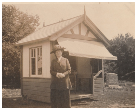
Turnabout on site August 1922
