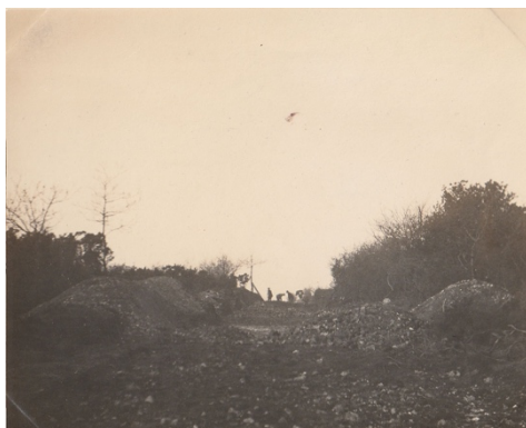
Cutting out the New Road March 1922
