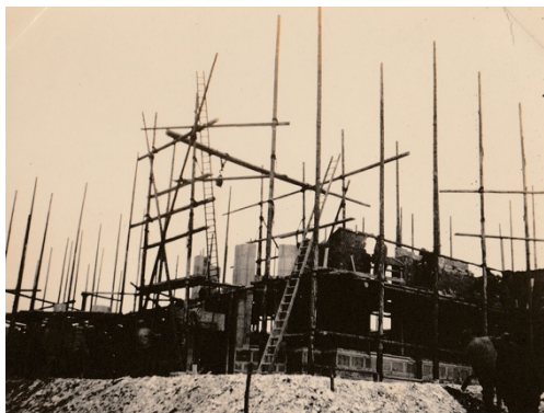
Raising first big Bay Window headstone, Drawing Room SW Corner
