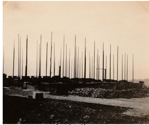
Front door side November 1921
