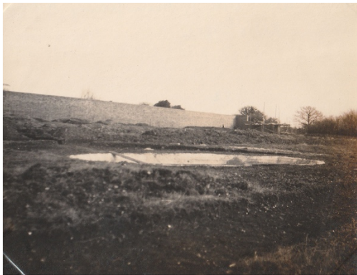
Pond and return wall by Maing Gateway Kitchen Garden December 6th 1922
