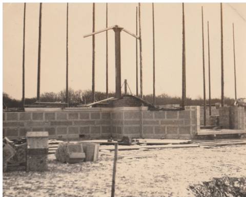
Lower stone plinth, West Side November 1921
