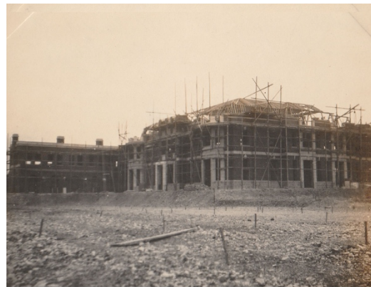
Skeleton of roof, from S.W. corner of tennis courts December 6th 1922
