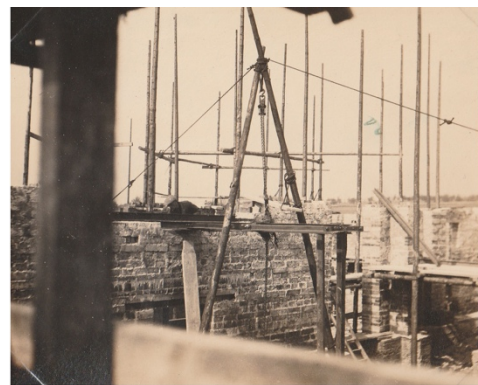
Iron girder in place for centre staircase platform March 15th 1922
