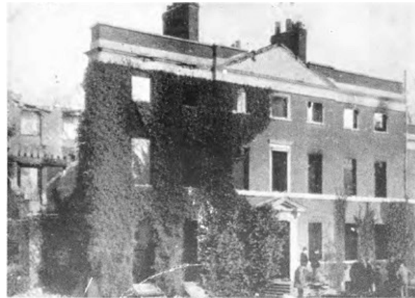
FIG 10a. Entrance to Westbury House after the fire
