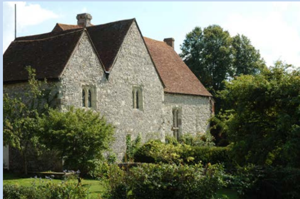
Figs 17 & 18 Exteriors of the Hall at the Court House, from east and west.
