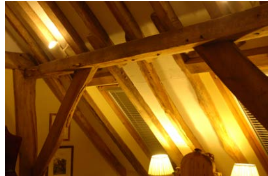
Fig 43. Roof of third bedroom
