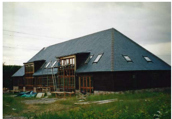
Fig 38. The new house nearing completion
