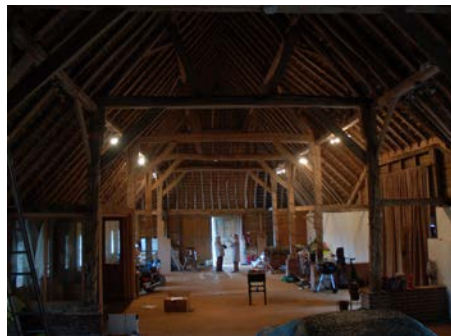
Fig 45. Interior Upper Parsonage Barn
