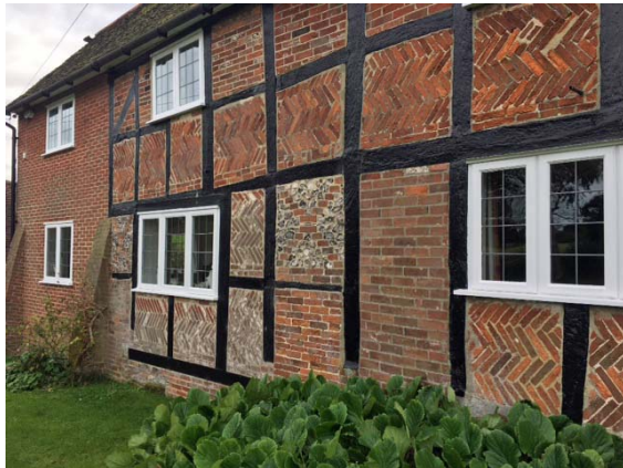
Fig 6. The central section of the house at Fishponds, the herringbone brickwork probably dating from the 16 th century and its occupant must have been a yeoman farmer .
