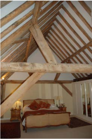
Fig 41 Tie beam and queen strut in second bedroom
