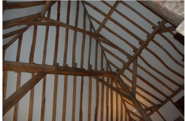
Fig 40. Ceiling of today's sitting room, showing collar above tie beam and purlin
