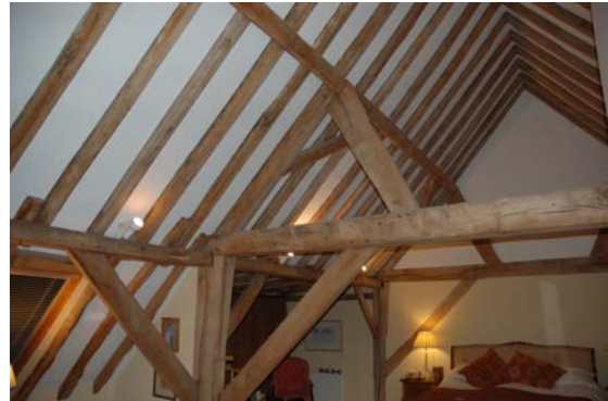
Fig 42 Ceiling of second bedroom
