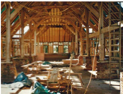
Fig37. Interior under construction
