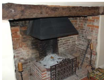
Fig 9. Fireplace in the original kitchen where family and servants
