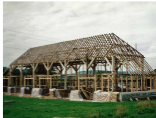
Fig 36 The framework of the old barn
