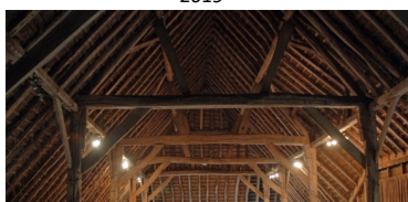
The restored beams and pillars of Upper Parsonage Barn
