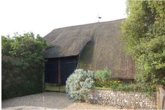
(Fig 2) The 17 th century barn at The Court House, which probably replaced an earlier barn for the collection of crops harvested for the rectorial tithes.
