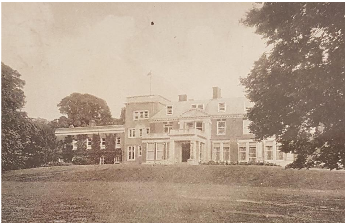
Figure 4: Westbury House rebuilt c1904-6 (photo taken early after re-construction) – north elevation
