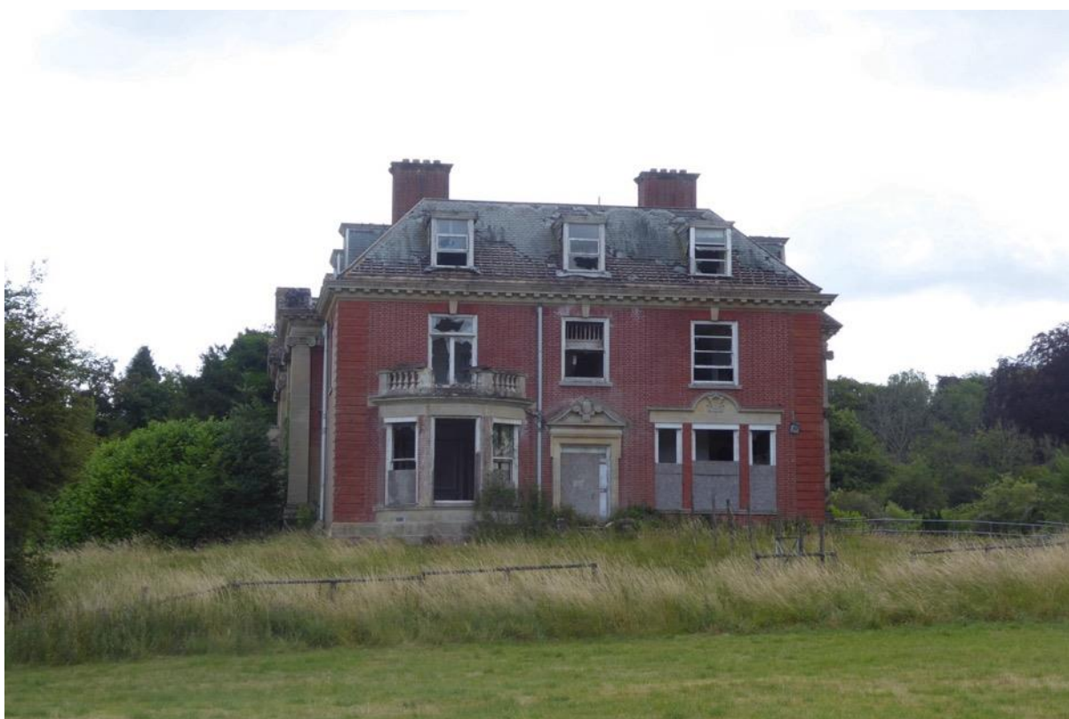
Figure 3: Westbury House – west elevation
