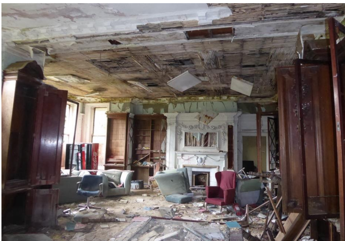
Figure 11: Typical internal finishes and condition of principal rooms to main house
