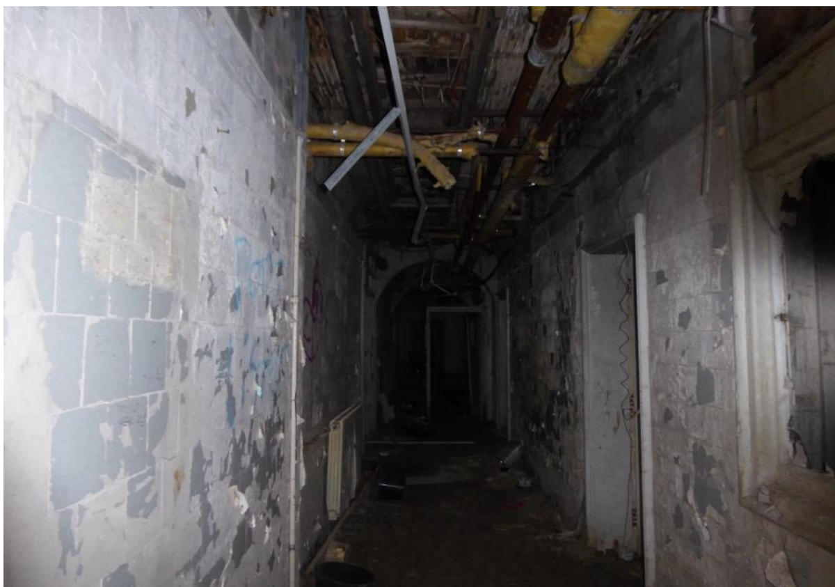
Figure 14: Lower ground (basement) 190406 main house- central corridor looking west
