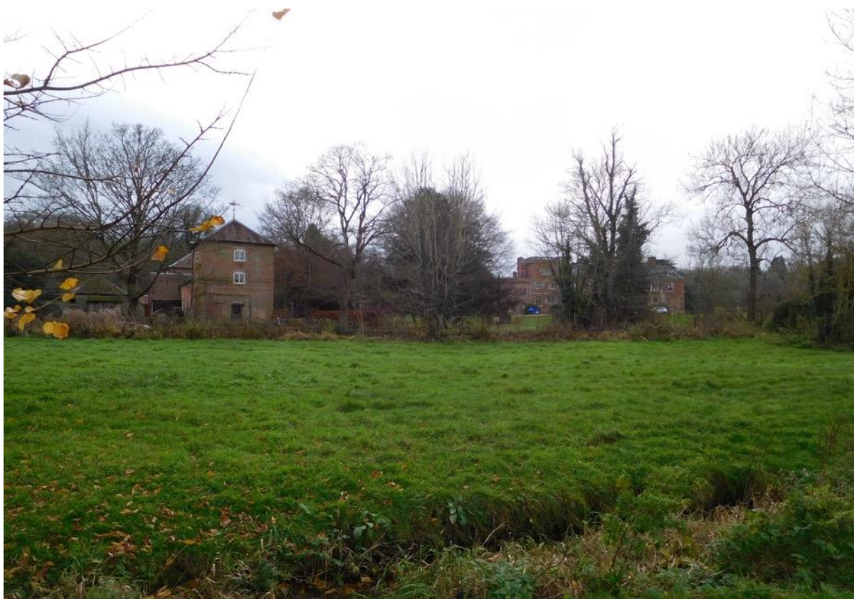
Figure 18: The former stables and coach houses from the north with Westbury House
