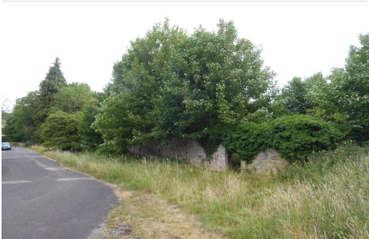
Figure 21: Walled garden to east side of access drive to Westbury House
