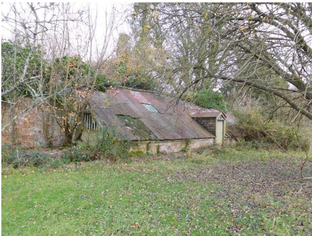
Figure 22: Late Victorian glasshouse to the northern boundary of the walled garden
