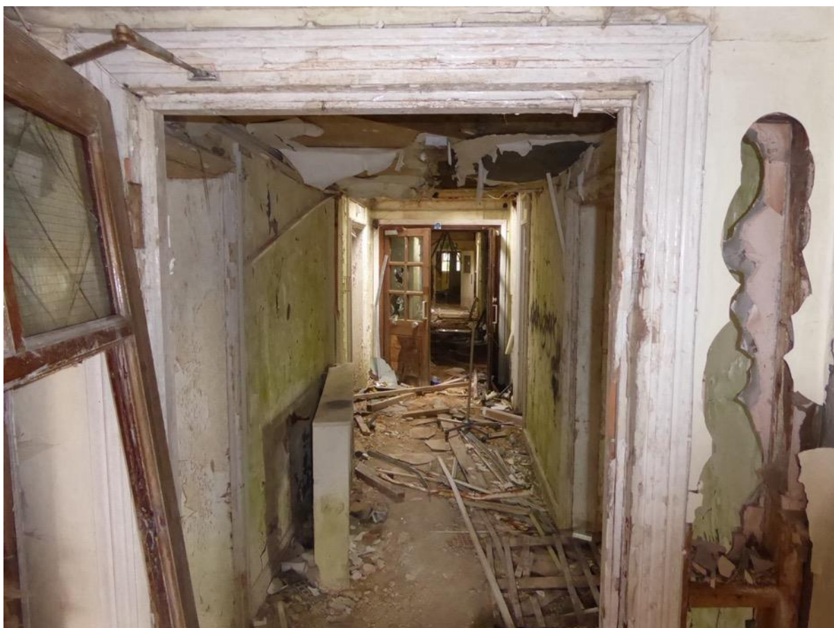
Figure 15: Lower ground (basement) looking east through late 18 th century wing
