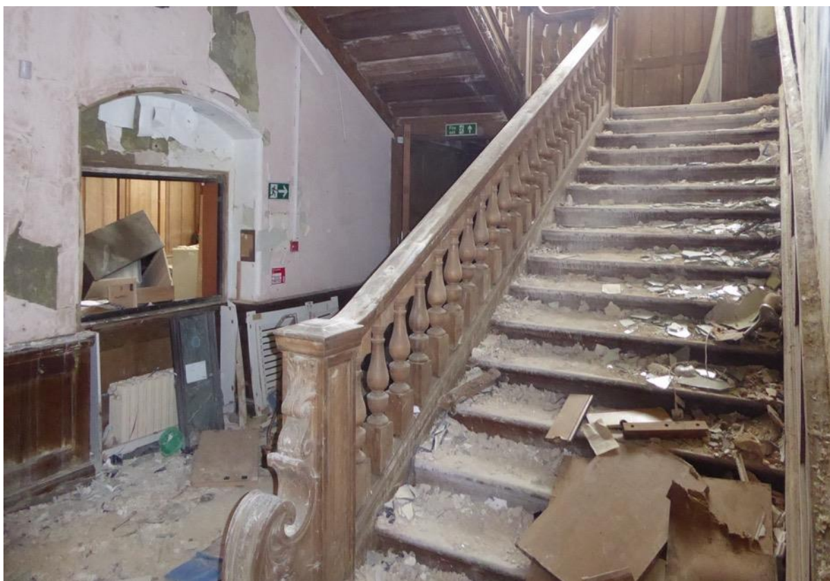
Figure 13: Principal stair ground to first floor
