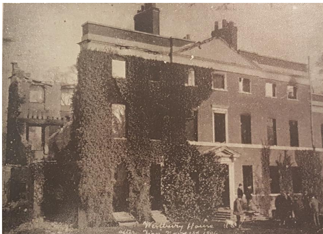
Figure 2: Westbury House immediate post-fire 1904 – South elevation
