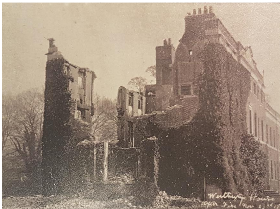
Figure 1: Westbury House immediate post-fire 1904 – west elevation (and part south)
