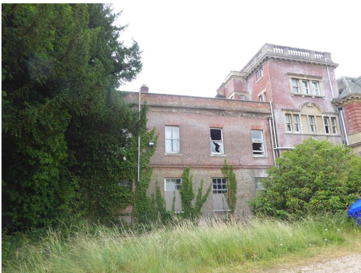
Figure 4: Late Georgian wing to the east of the 1904-6 reconstructed house
