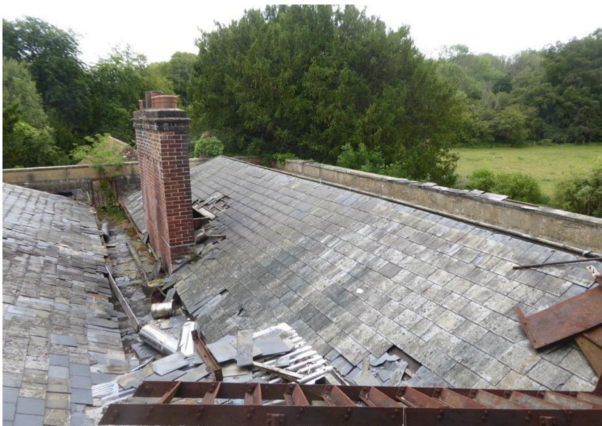
Figure 5: Roof of late Georgian extension
