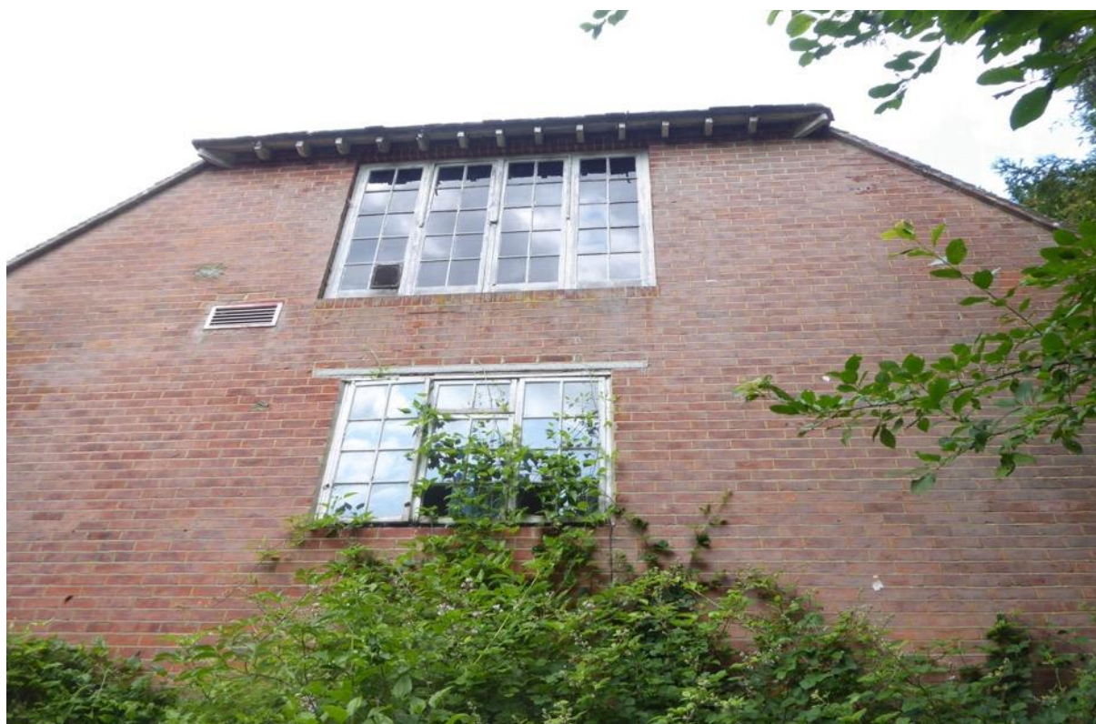
Figure 8: Late 20 th century wing extension to the east – east elevation with large half-hip
